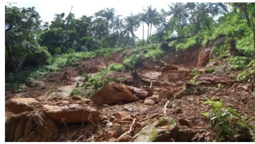
Figure 6: Crown of the debrisflow in Arthala estate
